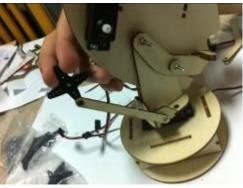
Then, connect the bigger hole to the screw at the neck's bottom. Tighten with a nylock locknut (leave option for some mobility). You may also tighten with a regular locknut. Place the cross on the servo and tighten using a bug screw.
